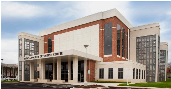
Iredell County Detention Center in North Carolina.
